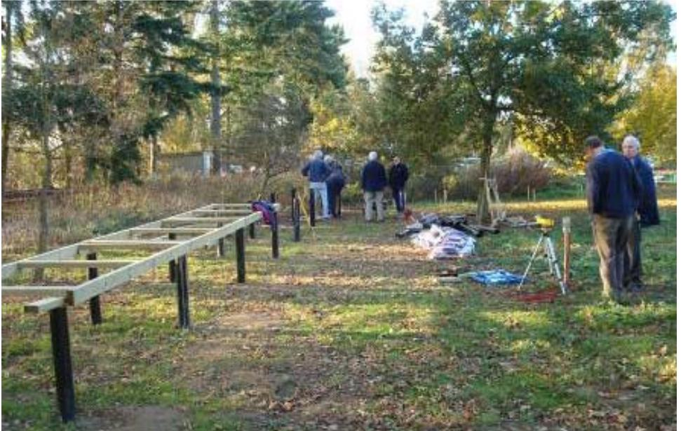
Main straight taking shape, Matt & Peter with laser level to left (on datum point). Track support frames just rested in position.
